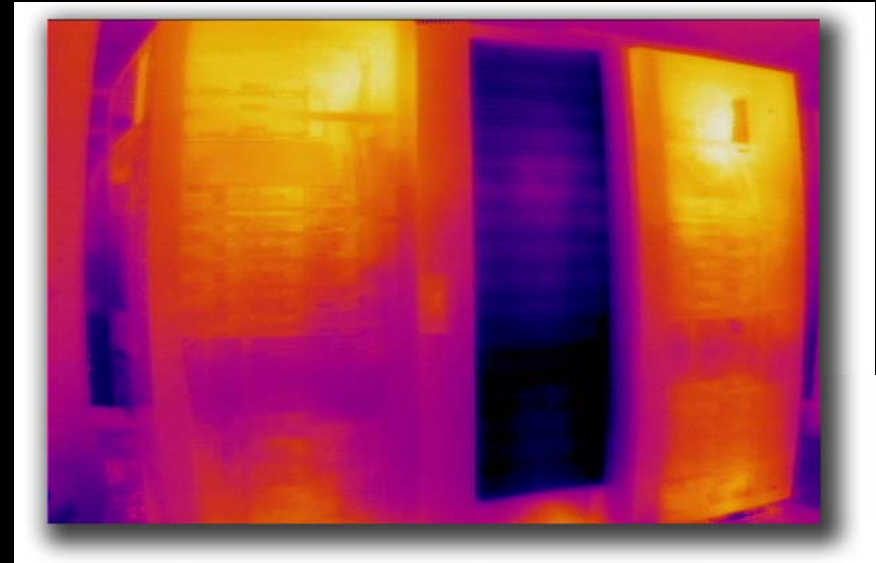
Thermal images of the Rear Door Heat eXchanger
